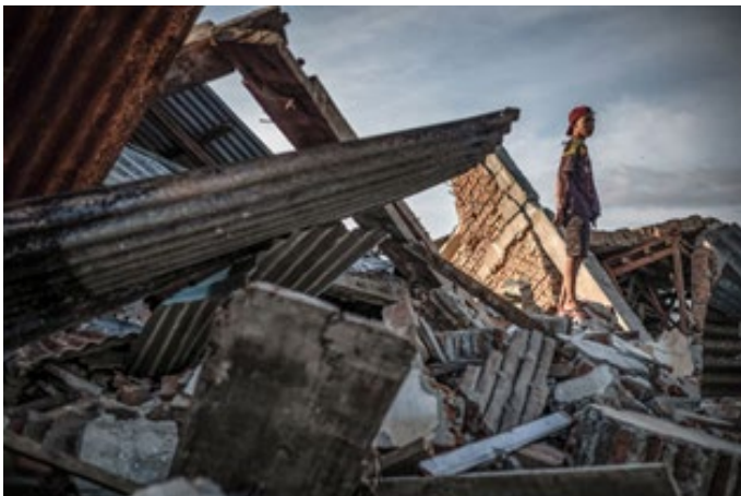
A collapsed building in the city of Palu in Sulawesi, Indonesia, after a magnitude-7.5 earthquake hit the region in September 2018.
